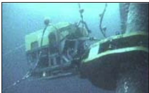
Figure 5.3. Abrasive waterjet cutting. Presentation for the Oil and Gas UK decommissioning seminar 12 June 2008.
