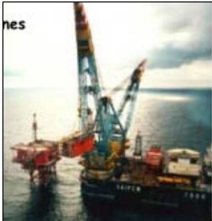
Figure 5.2. Removal of topside from Odin platform. The 7,700 tons topside is lifted module by module. Source: Kirsting (Aker Solutions). Presentation for the Oil and Gas UK decommissioning seminar 12 June 2008.
