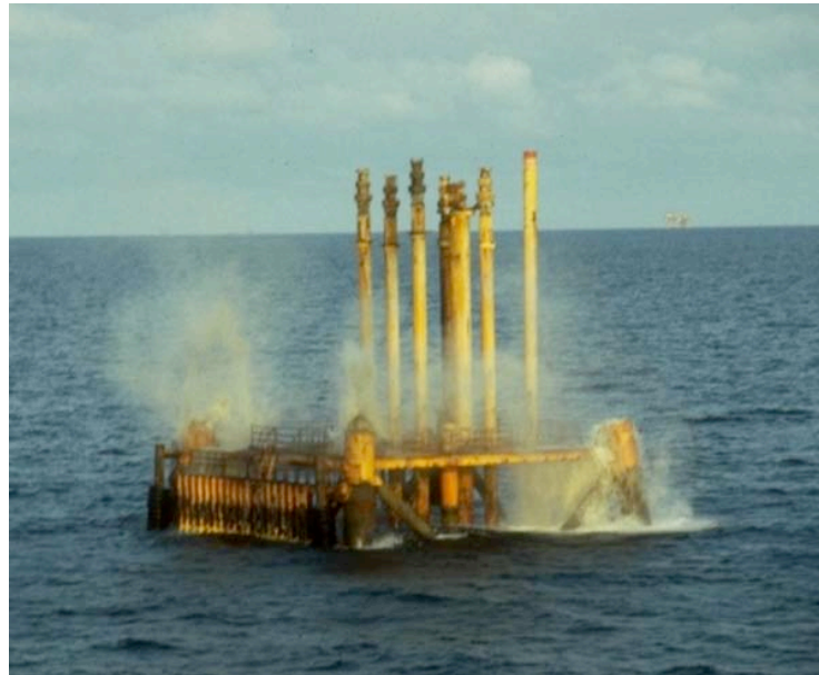
Toppling involves explosives to sever the base of the structure below the mud line. Photo: Louisiana Department of Wildlife and Fisheries
